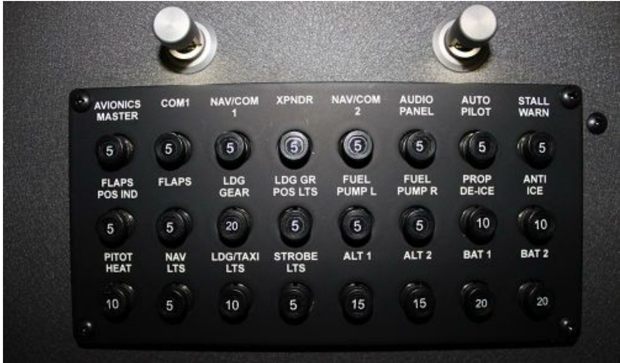
Circuit Breaker Panel
